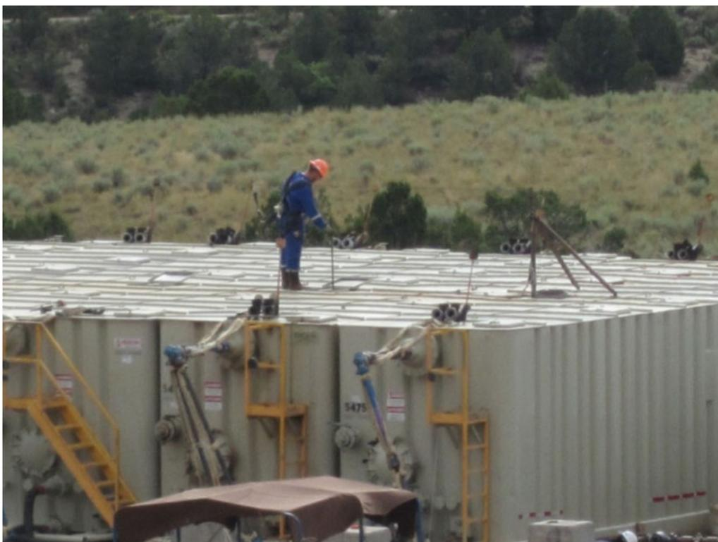
**FIGURE 2.** Flowback technician gauging a flowback tank. (color figure available online)
