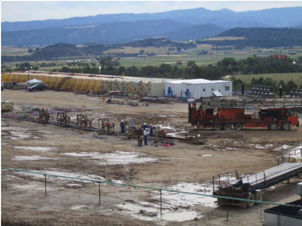
**FIGURE 1.** Well site with flowback tanks. (color figure available online)
